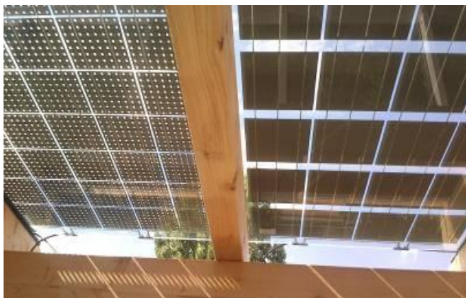
Fig.1: Semi-transparent or opaque (light-impermeable) PV cells
