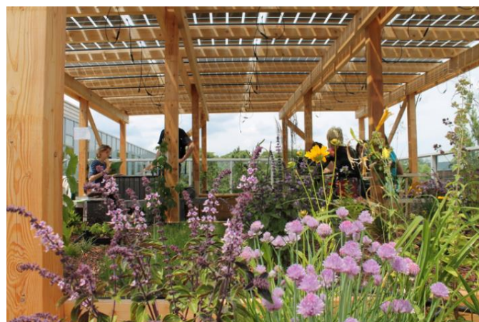
Fig. 2: Habitat with bifacial PV, wooden substructure and plants, realization ATB Becker GmbH
