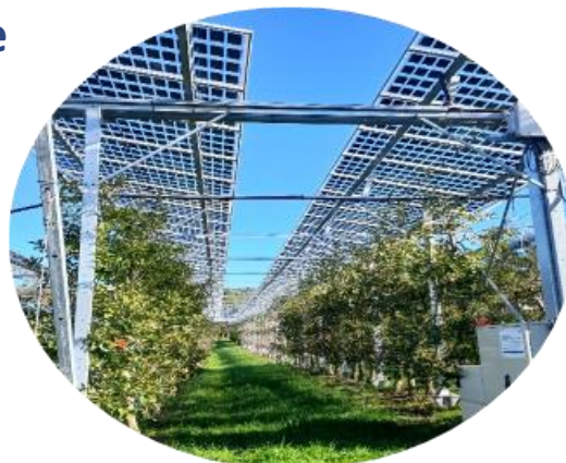
Figure 1: High elevated system with continuous row of modules - Experimental station for fruit and vine cultivation in Haidegg.
